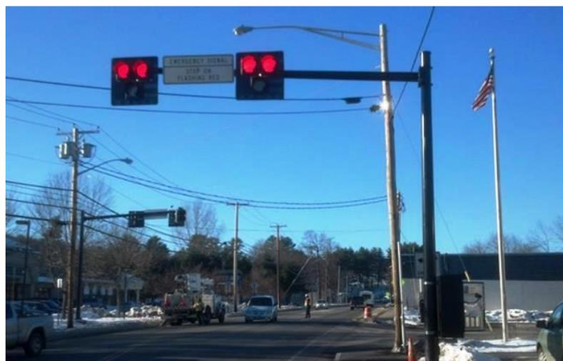
The city's first Emergency Vehicle Hybrid Beacon. The flashing sequence is activated for fire trucks leaving Central Station on North State Street.
