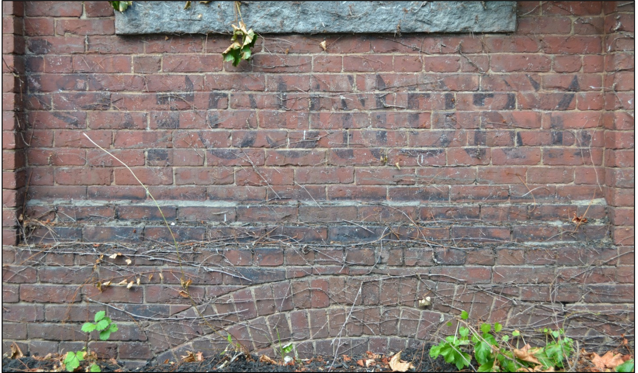
Top of arched tunnel (filled) leading under the 1881 wing to the Ford & Kimball Foundry
