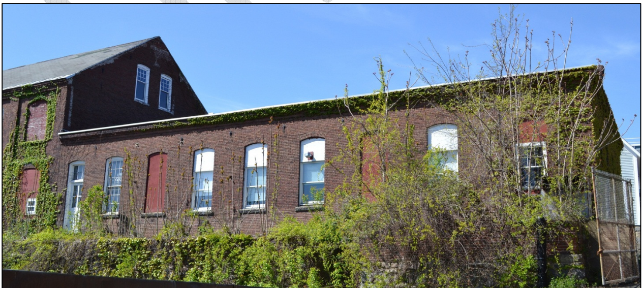
Eastern elevation of the 1881 wing, without wall buttresses defining window bays.
