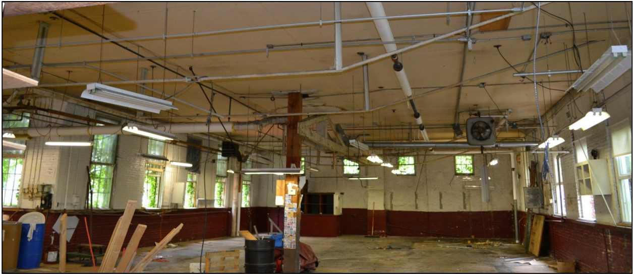
Interior, one-story leg of 1881 additions, looking north, showing metal queenpost trusses supporting the roof system.
