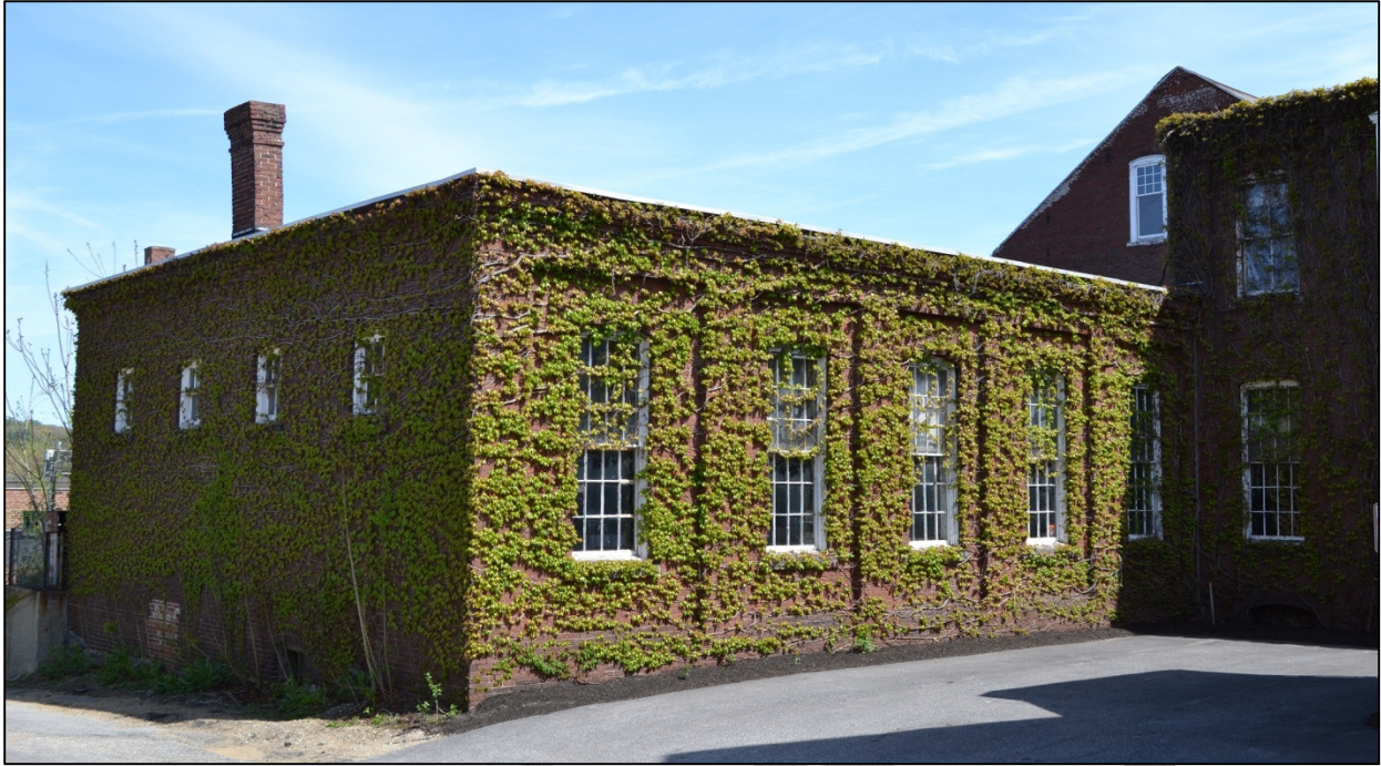
North (end) and western elevations of the 1881 wing, built as a machine shop extension, showing wall buttresses defining window bays.
