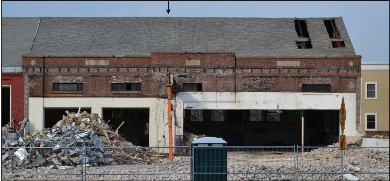
45 South Main Street during demolition, 2012, following the removal of a later addition at the front and revealing the façade created in 1932. The roof of the former engine house was raised in 1932 to the elevation of the roof of the original shop building of circa 1866, and a new façade of brick laid in Flemish bond was applied across the altered buildings (note central date tablet). The arrow indicates the juncture of the original roof (right) and the raised roof (left).
