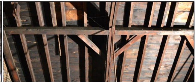
Right: Western roof of the southern building, seen from below. Former scuttles in the roof are indicated by irregular rafter placement and lighter-colored sheathing.
