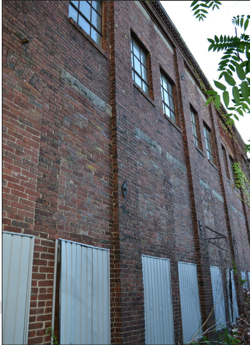
Eastern elevation of southern building, showing evidence of original window openings, lintels, brick piers between windows, and wall buttresses defining bays for pairs of windows.
