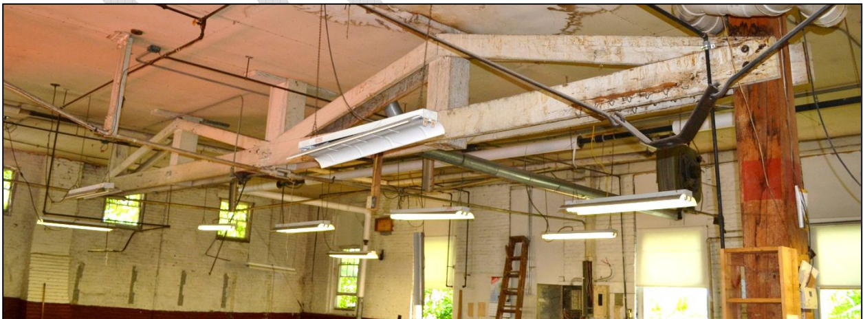
Timber kingpost truss system added to the metal roof trusses of the one-story leg of the 1881 addition and resting on the bottom chords of the metal trusses except at far right.
