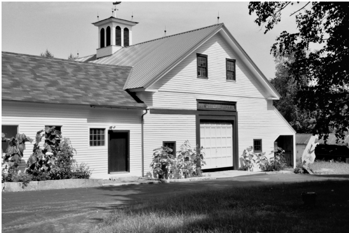
Photo 3 description: Front (south) elevation of barn and east end of attached shed Roll: 4 Frame: 8 Direction: NE
