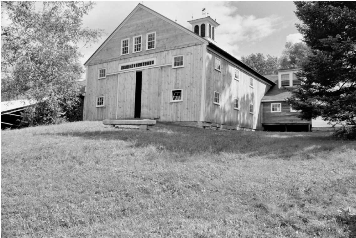
Photo 5 description: Rear (north) & west elevations of barn and rear of shed (east end) Roll: 4 Frame: 12 Direction: S
