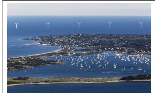
Block Island Wind Farm, Rhode Island
